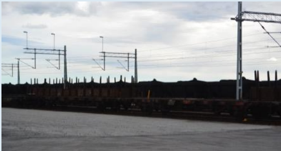
PUBLIC ACCESS ELECTRIC RAIL
