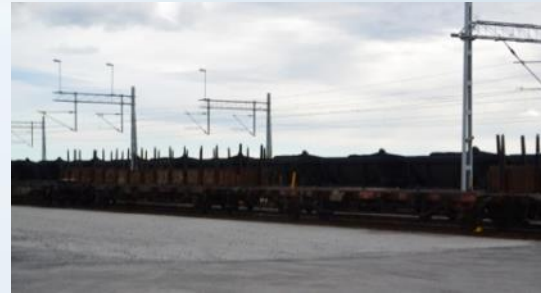
PUBLIC ACCESS ELECTRIC RAIL
