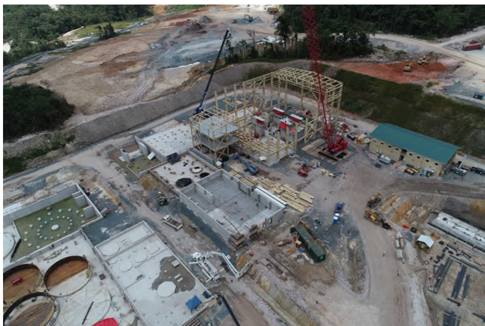
Figure 12: Fruta del Norte process plant under construction , December 2018
