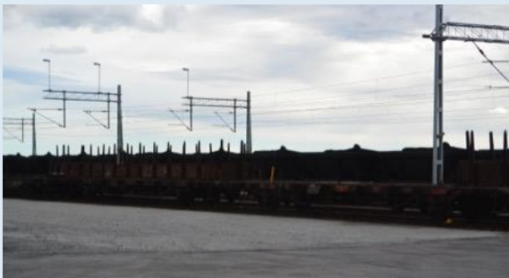
PUBLIC ACCESS ELECTRIC RAIL
