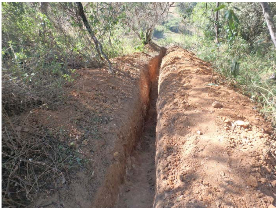
Photograph of completed trench. Samples are collected from basement rock either by continuous rockchips or by diamond saw cuts, and sampled to geological boundaries
