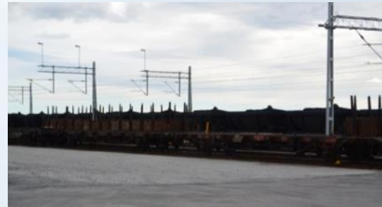
PUBLIC ACCESS ELECTRIC RAIL
